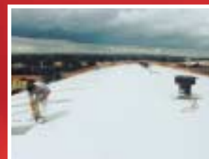
A corrugated metal roof protected from ongoing corrosion with Corro-Tech GP and Uni-Tech UV.
