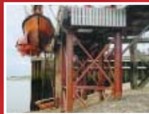
Offshore training rig supports coated with Chemi-Tech UW, a corrosion resistant lining for underwater environments.
